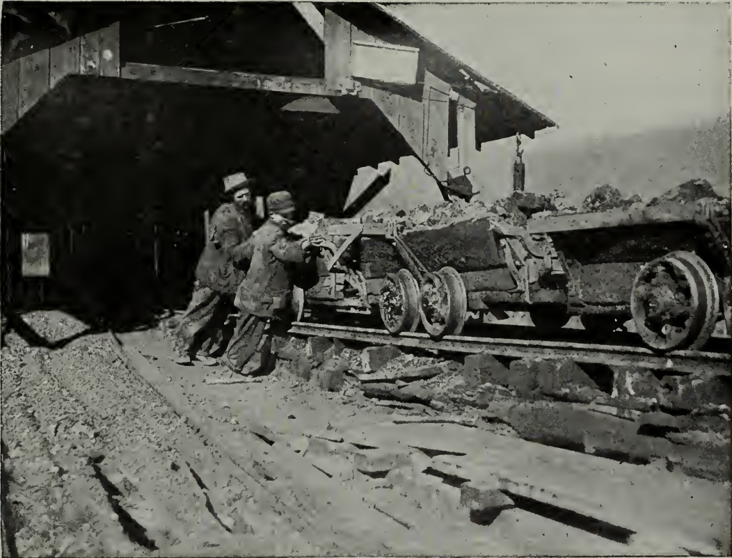
FIG. 62.—Shoving Cars in a Coal Mine.
